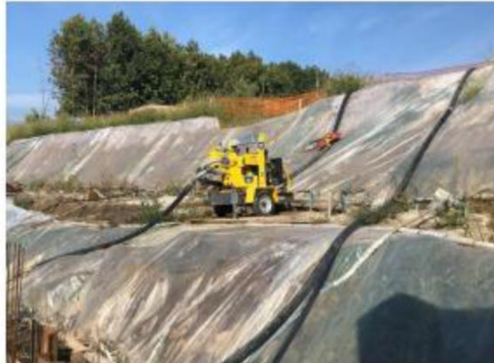
Well point – WEL ECO (Tunnel Construction)
